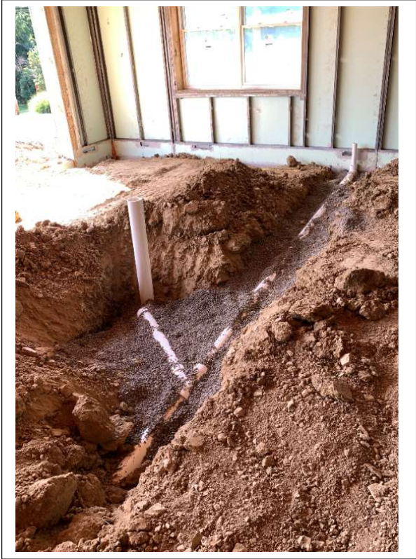
The plumbers installed drains into the garage
